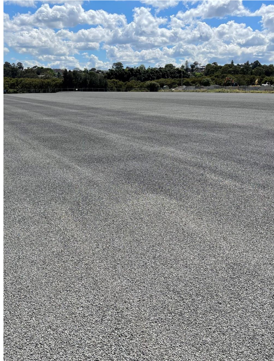
Figure F2. View of site facing northeast.
