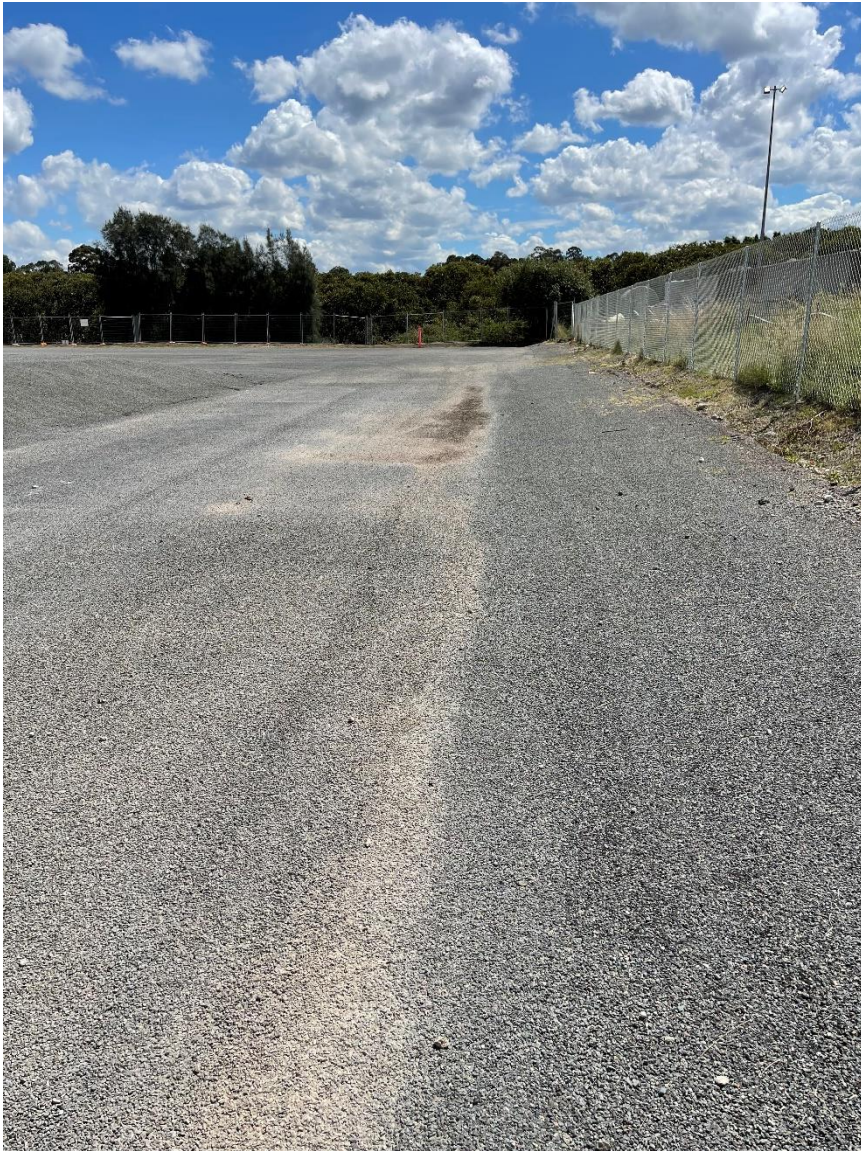
Figure F5. View of eastern boundary facing north.
