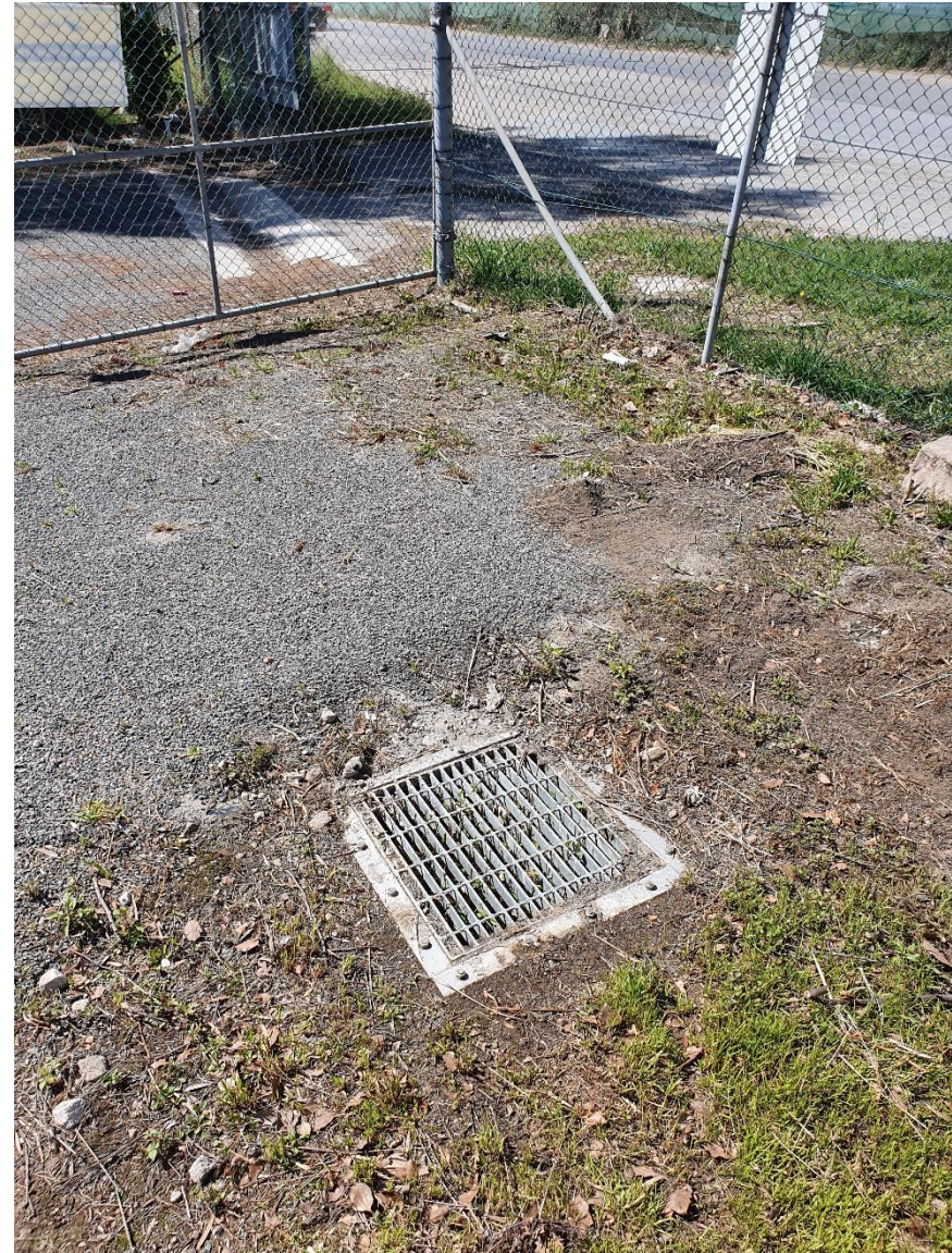
Figure F4. Stormwater drain pit along the front boundary of the site.
