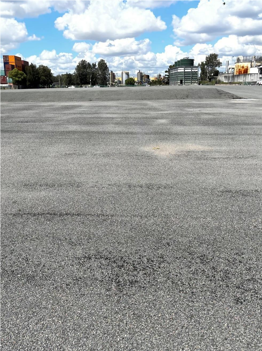
Figure F1. View of site facing south showing capping layer.
