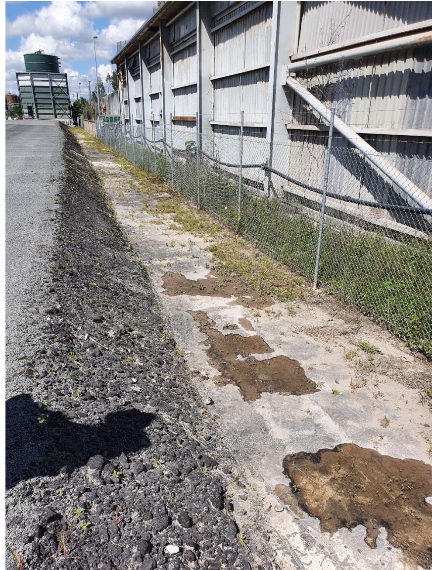
Figure F8. Capping seal along western batter.
